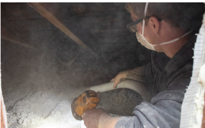
Above: Weatherization staff use various ways to determine where air leaks could be in the home. Below: Weatherization staff install insulation in an attic.
