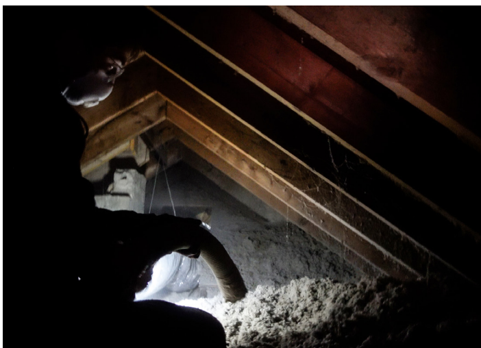
Crew Leader Kyle Paulsen installing insulation in the couple's attic
