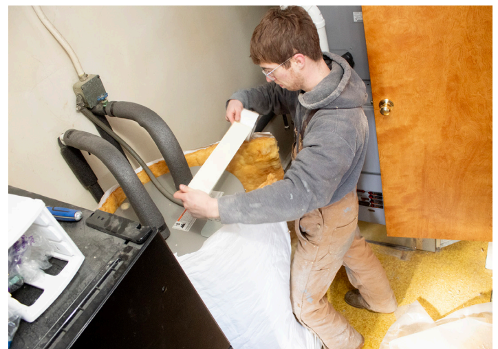
Crew Leader Kyle Paulsen installing a water heater wrap
